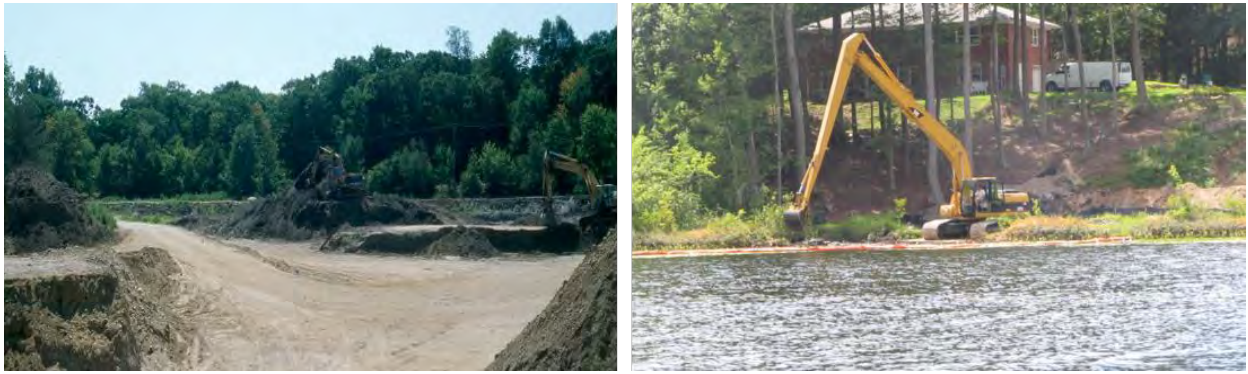
Figure 13. Dry dredging (left) and wet dredging (right)
